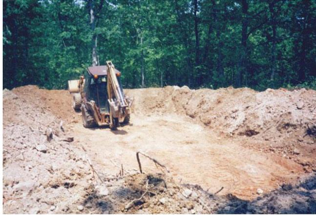
A septic lagoon, of adequate size of course, is probably the simplest system to use and maintain. Because of its large size, solid buildup on the bottom is very slow. An oversized lagoon may never need to be pumped out during the lifespan of the house using it.
